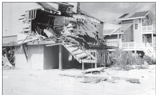
Figure 2. Well-sited building that still sustained damage.
