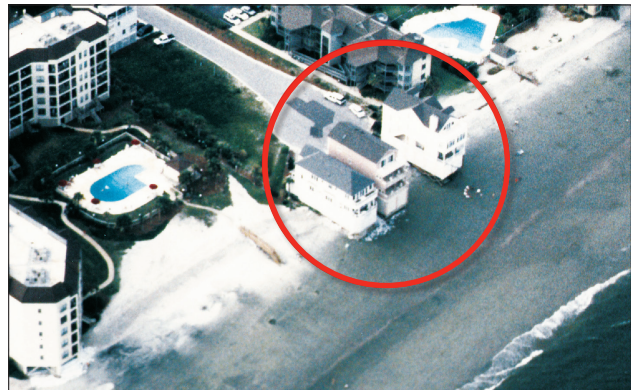
Figure 1. Well-built but poorly sited building.
